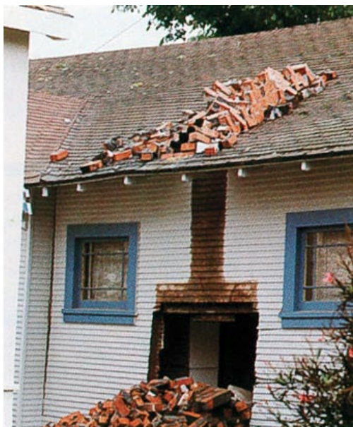
Failed masonry. Before this chimney collapsed, it first snapped at the roof line.
