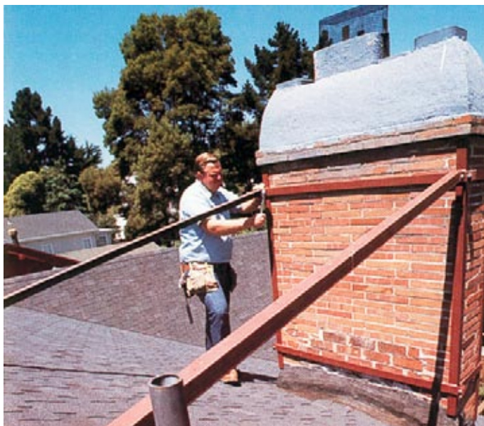
Steel frame. Braced chimney has a collar to hold it together and braces to keep it from coming down.
