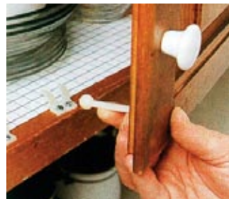
Cabinet doors. Install child-safety latches on all cabinet doors to prevent contents from falling out.
